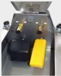
Photo with additionally installed low pressure float valve (yellow)
