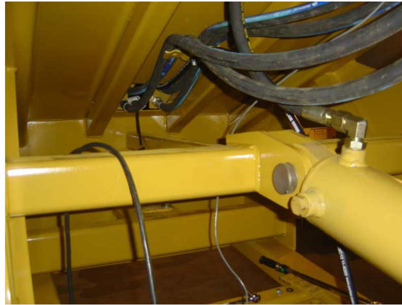
View of the tandem hose routing, the push off framework and push off cylinder.
